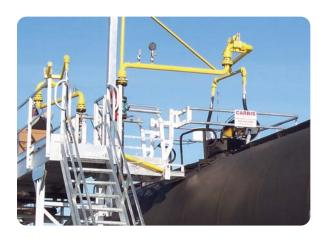
There are several arm designs that can be tailored to specific needs. Top loading arms include single arm fixed reach, scissor type, supported boom and unsupported boom. Bottom loading arms, which are the preference in the industry, have similar designs including an unsupported boom, A-frame, A-frame spring balanced and counterweighted. Marine loading arms load/unload barges and carriers.
