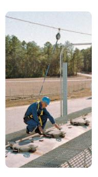
fall arrest system. A fall can turn into an emergency situation quickly. When a worker has fallen, they may be unconscious, and there should be a rescue plan to bring the worker to safety quickly. There are a couple of major life-threatening syndromes that can occur after a fall. Harness hang is
